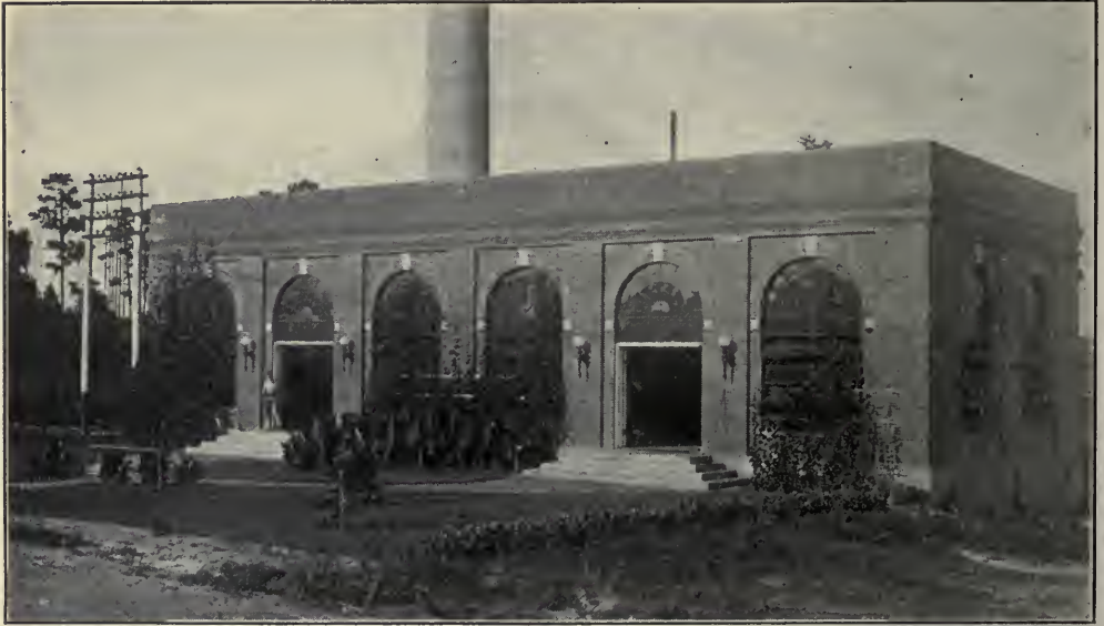
EXTERIOR OF THE GAINESVILLE, FLA., MUNICIPAL POWER-PLANT
